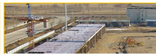
Zhangjiakou module Facility Hebei Province Under the construction
